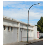
Pole street lighting (ToVP standard)
