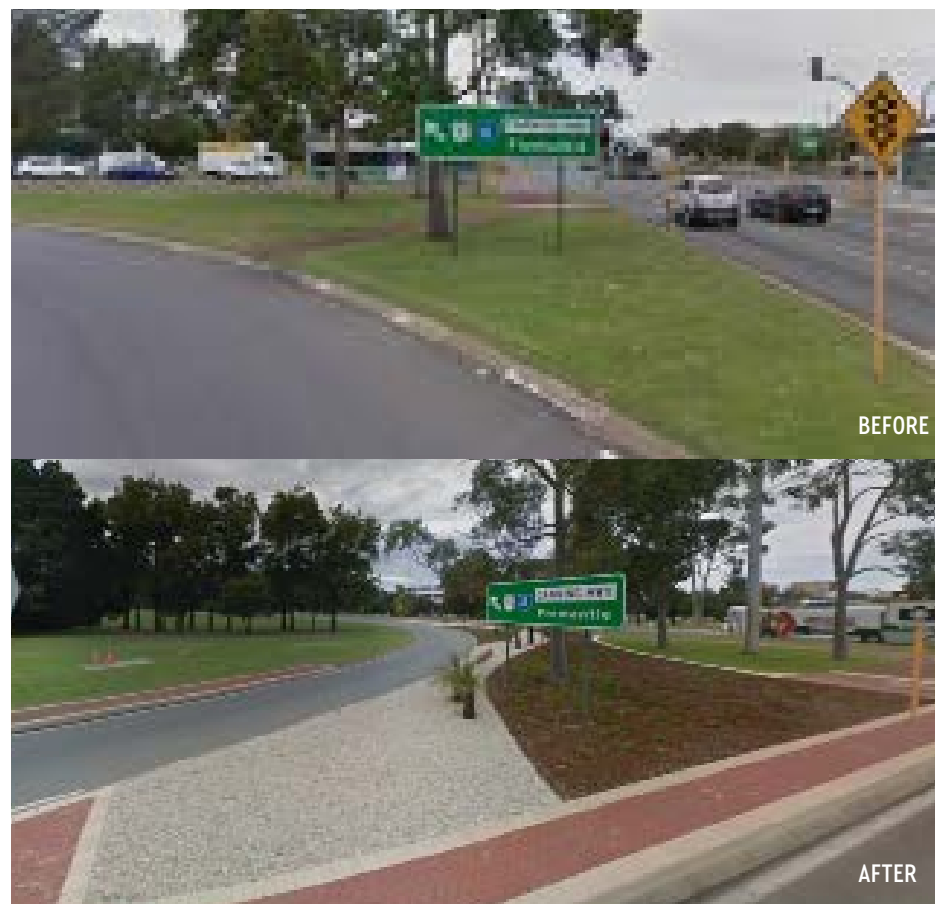
Image 9. Slip-road onto Canning Hwy from Albany Hwy
