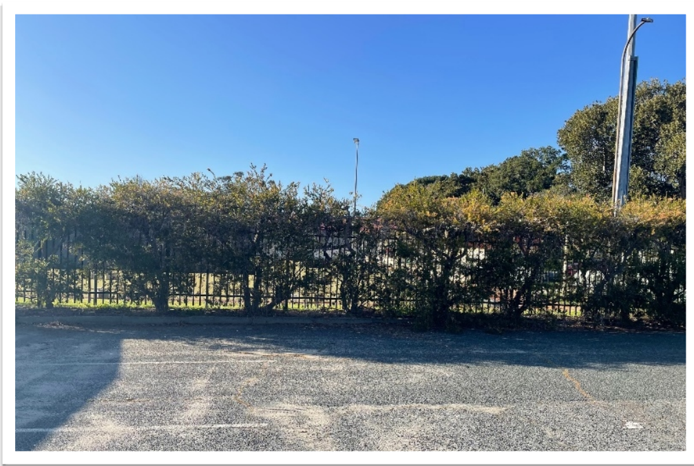
Fence installed by the Town. Photo taken from inside the Victoria Park Carlisle Bowling Club carpark.
