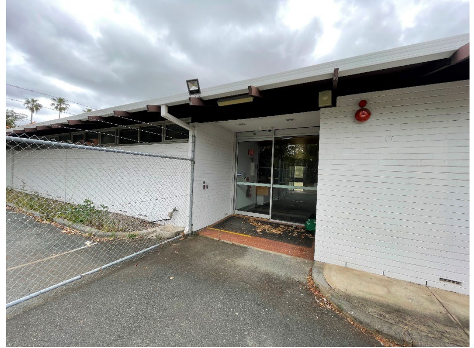
Figure 7: Sliding door entrance on south elevation
