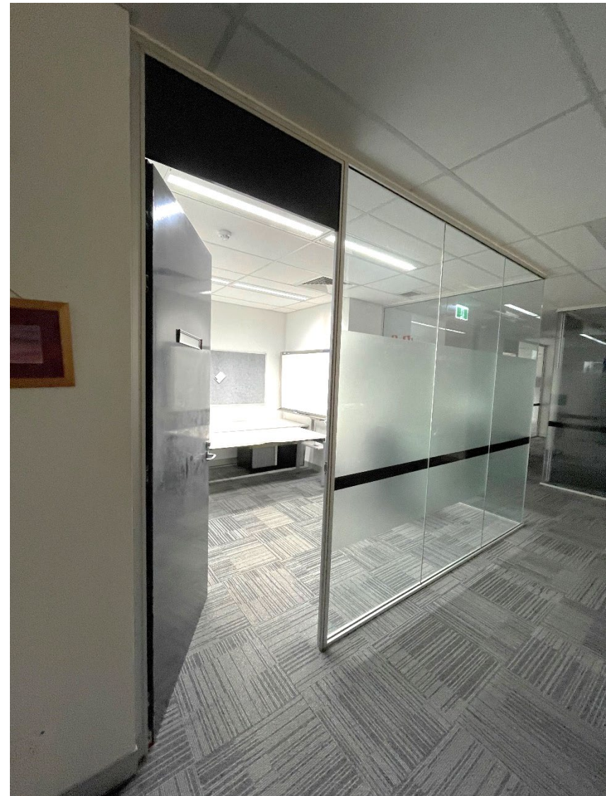
Figure 17: Glass partition walls
