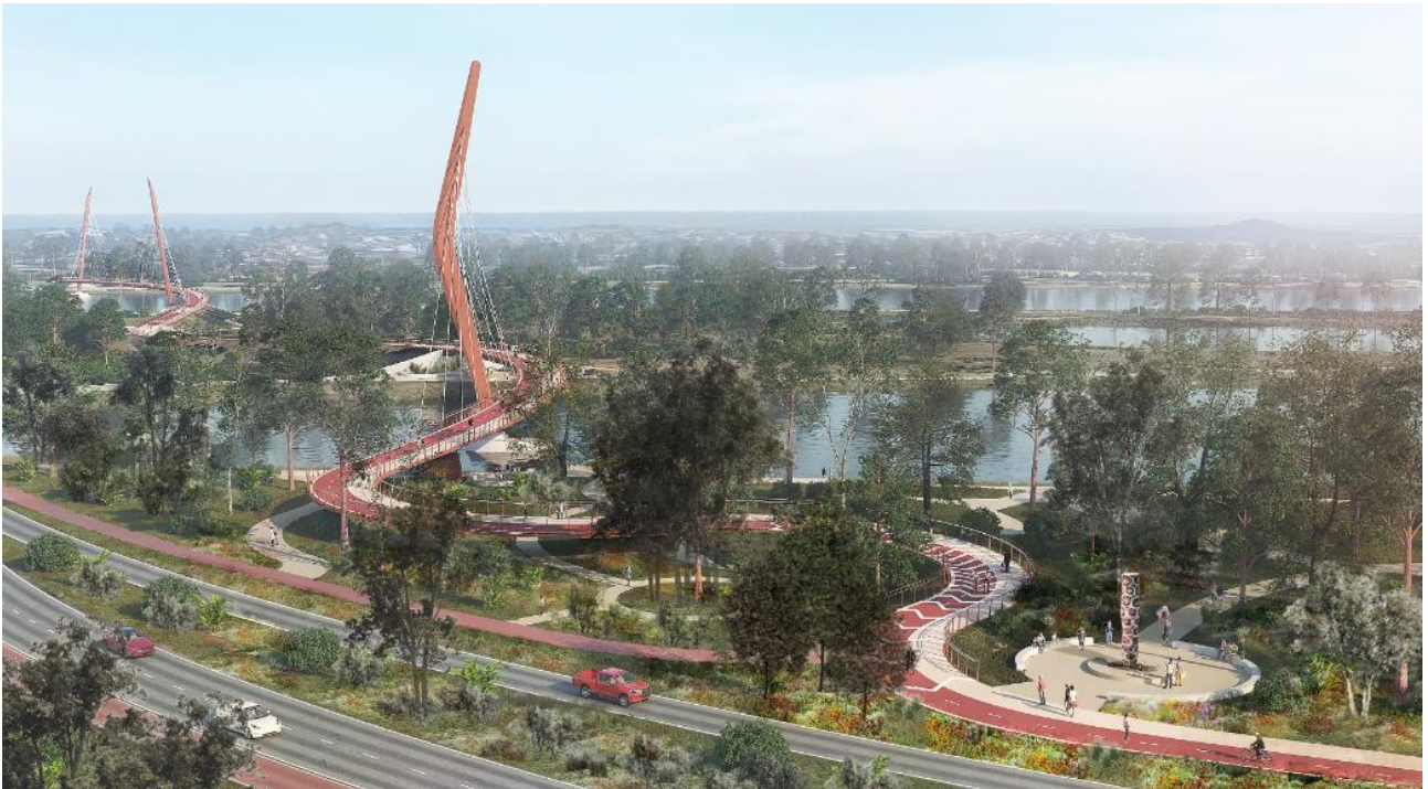
Figure 4-3 Proposed Bridge Construction
