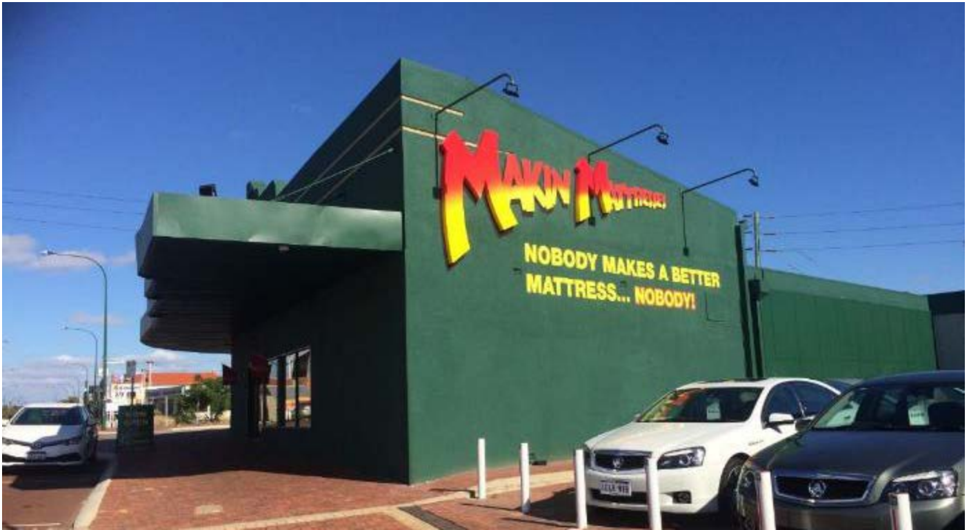
Figure 13: Signage to north elevation
