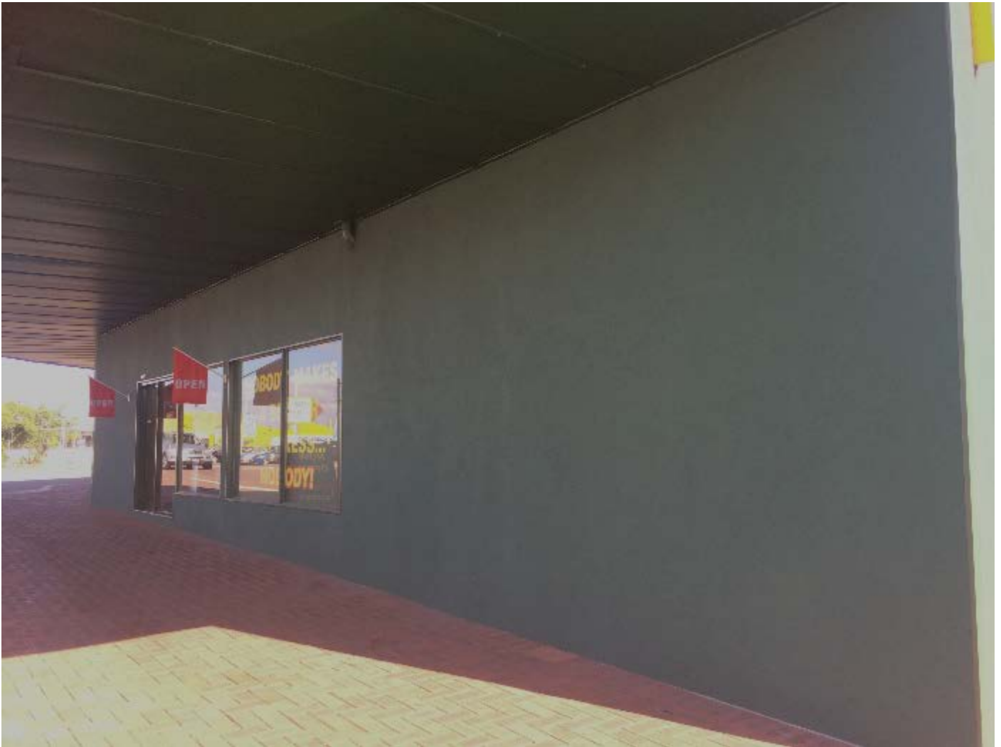
Figure 9: Blocked up windows to Albany Highway facade
