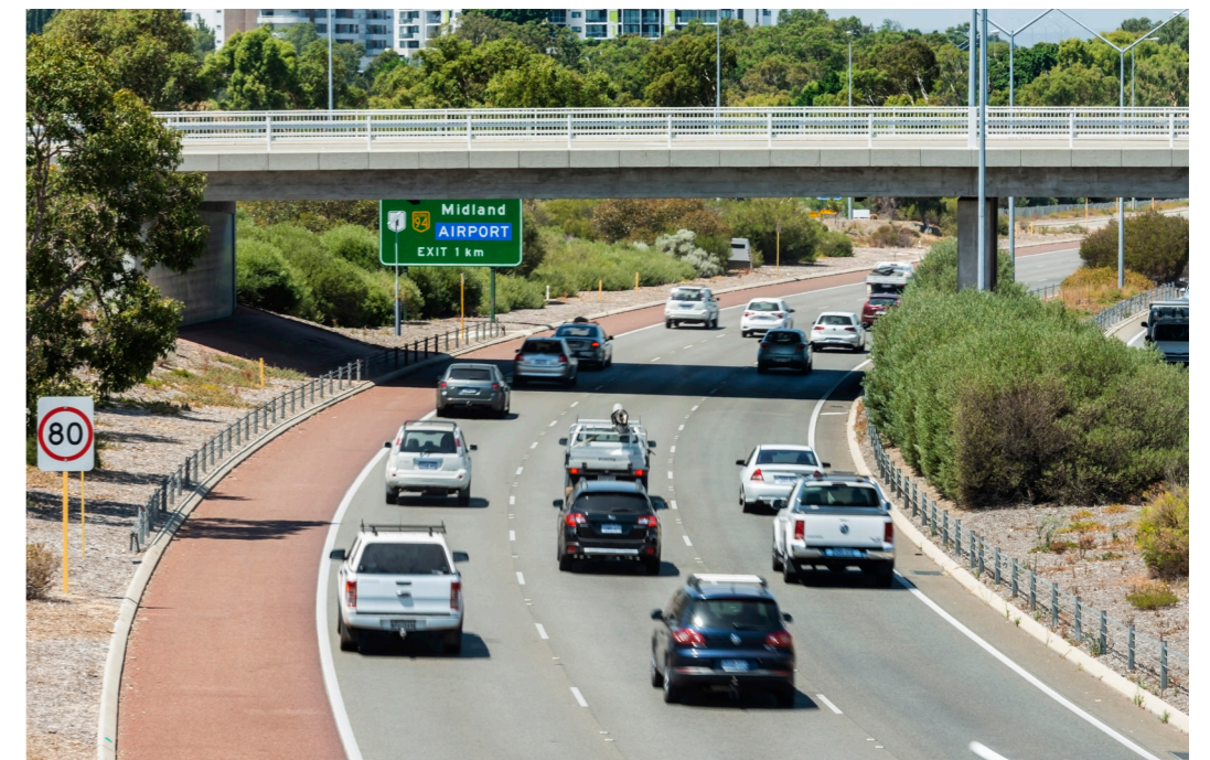
EXISTING CITY OUTBOUND VIEW
