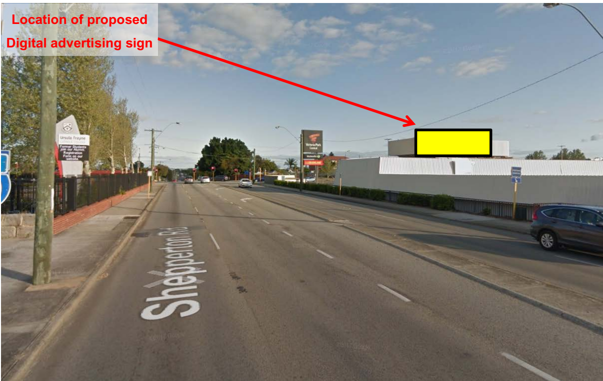
Figure 6-2 Close-up of Existing Visual Environment – Shepperton Road
