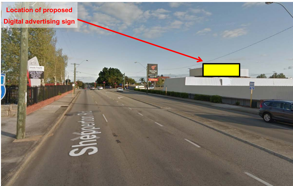
Figure 6-2 Close-up of Existing Visual Environment – Shepperton Road
