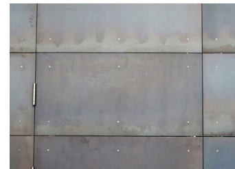
METAL CLADDING - EXPOSED JOINTS
