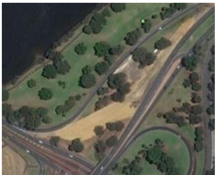
Following tree removal for new on-ramp December 2016
