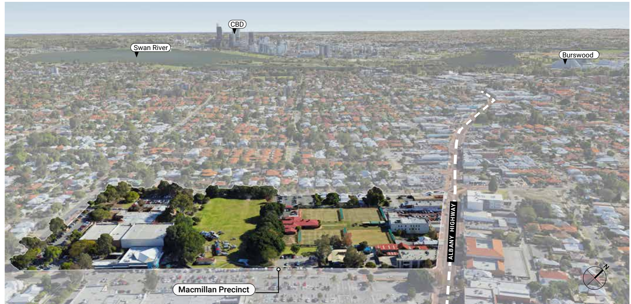
Views to Swan River, Perth CBD and Burswood | Macmillan Precinct
