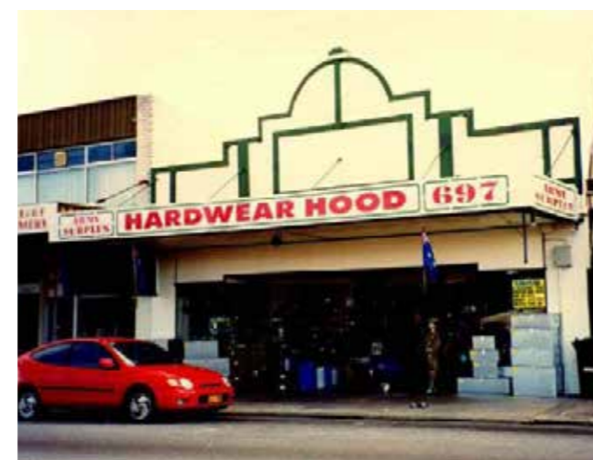
Heritage Listed Building (Town of Victoria Park 2000 MHI)
