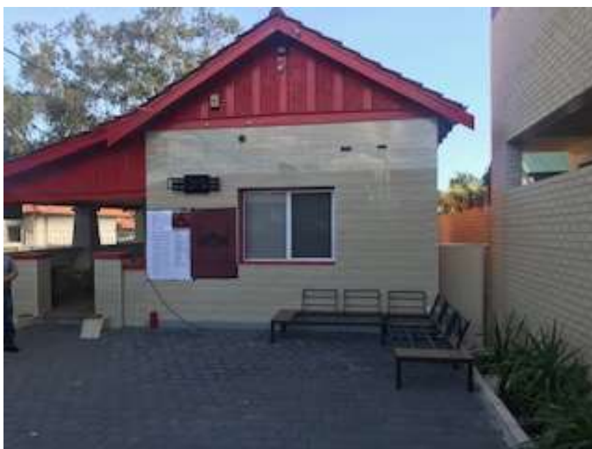
Picture 2 – Outdoor smoking area – Back corner and area to the right side of the picture is presumably the area that the smoke is travelling to the neighbour's property (the green roof)
