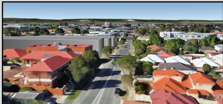
Figure 15: 3D perspective looking south-east along Swansea Street showing the scale of the proposed development in relation to the built form of the surrounding area with the Brightwater Oats Street aged care facility in the foreground.
