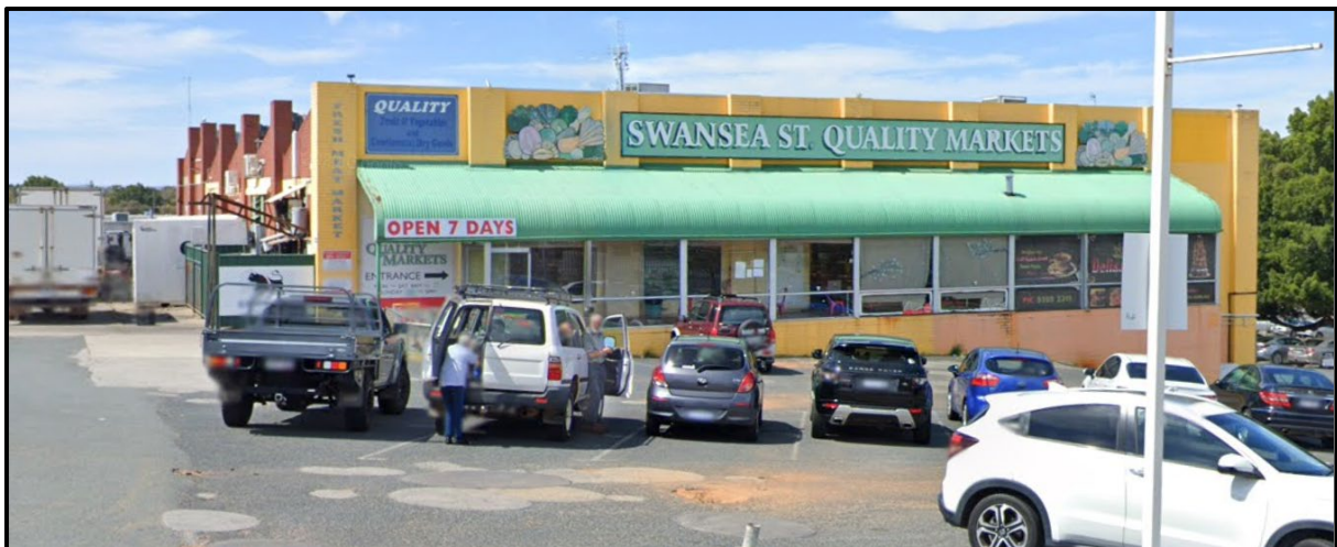
Photo 1 – View north-east from Swansea Street towards the Swansea Street Markets frontage
