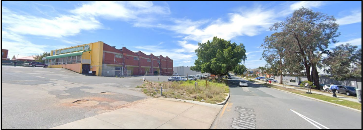
Photo 4 – View north from intersection of Swansea Street and Millford Street towards Swansea Street markets building
