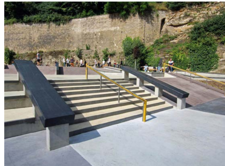
ADVANCED STAIR SET / RAIL / DOWN LEDGES
