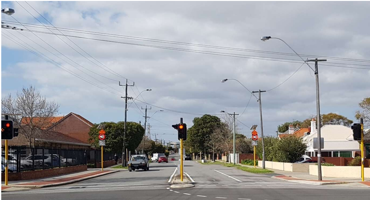
Photo 3: Short section of kerbed median on Duncan Street approach.
