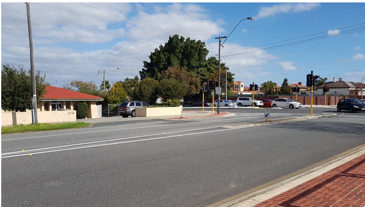
Photo 4: Duncan Street widening near the signalised intersection.
