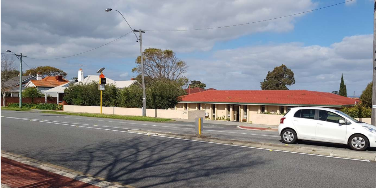
Photo 1: Existing single storey buildings on the site.
