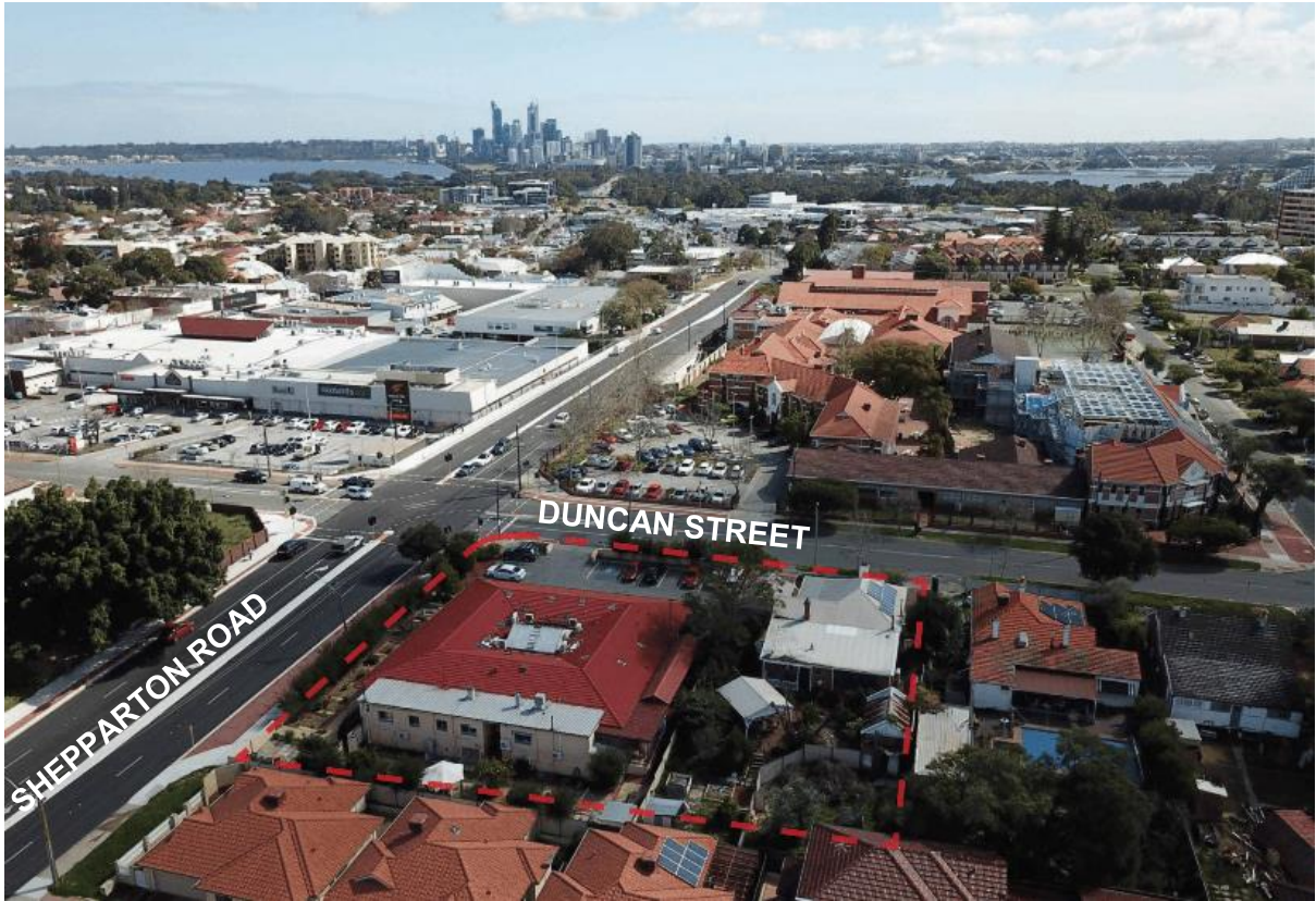
Photo 4: Aerial photo showing the entire subject site looking north-west towards Perth CBD.
