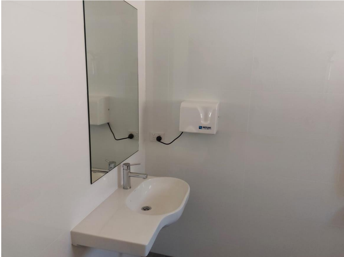
Image 7 – 10 Kent Street Universal Access Toilet
