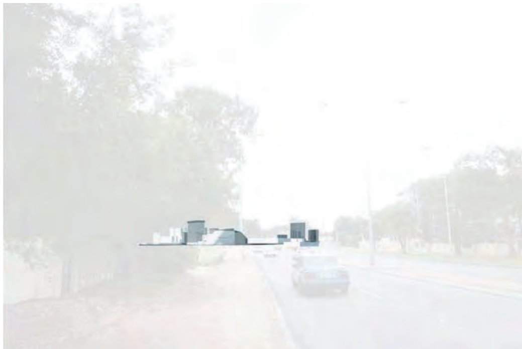
VIEW 7A: ("GHOST" IMAGE) - THIS VIEW DEMONSTRATES THE 'LOCATION' OF BURSWOOD LAKES IN VIEW 7. HOWEVER, THE DEVELOPMENT IS SCREENED BY EXISTING BUILDINGS AND MATURE TREES.
