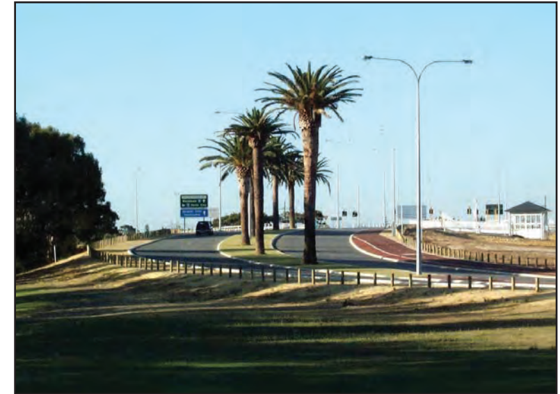
Burswood Link Road adjacent to Burswood Lakes site
