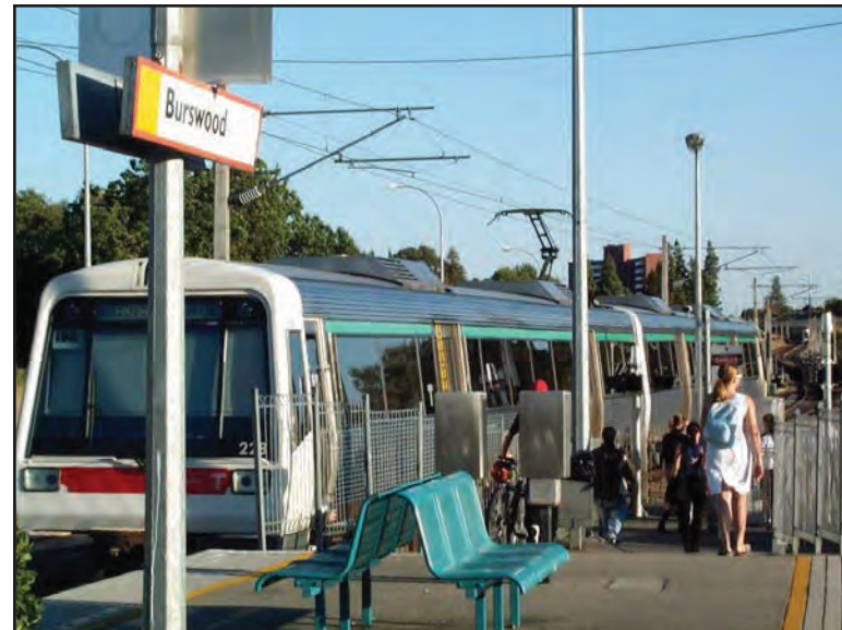
The Burswood Railway Station
