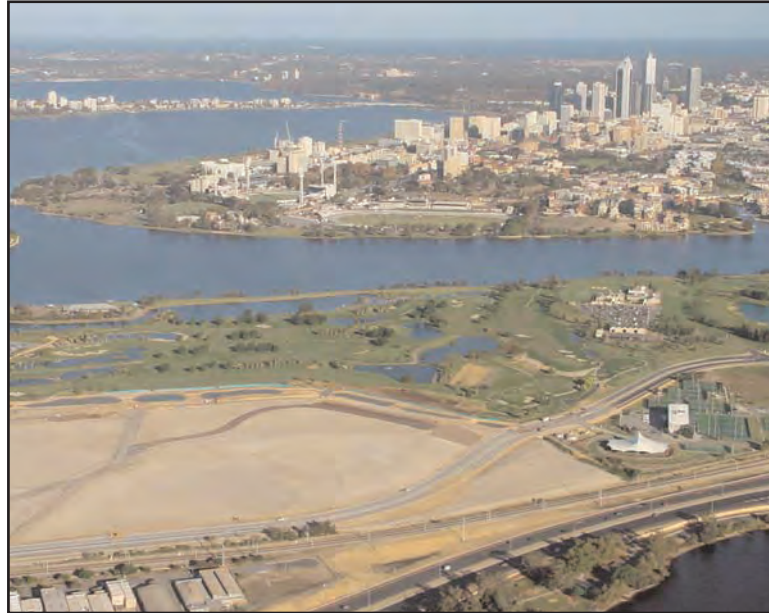
Aerial view of Burswood Lakes site looking west to the Perth CBD.
