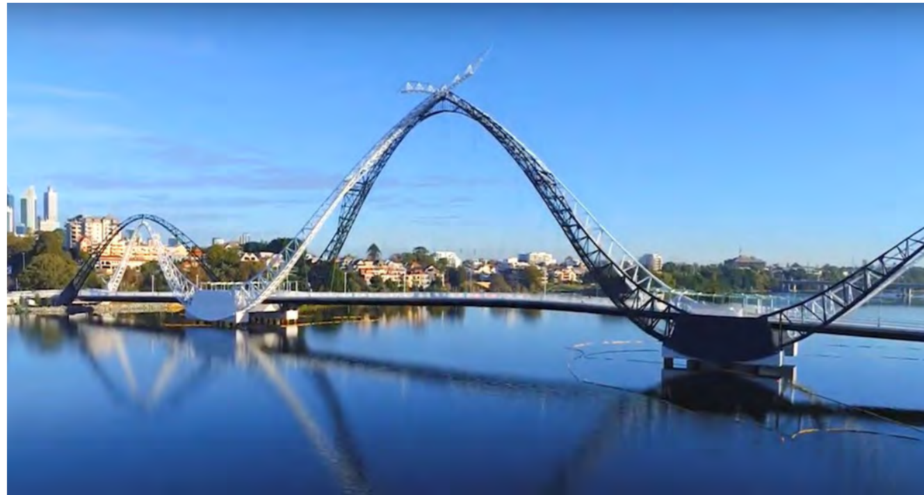
Matagarup Bridge to the west of the Structure Plan Area
