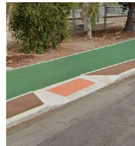
Align cross connectors with existing pram ramps
