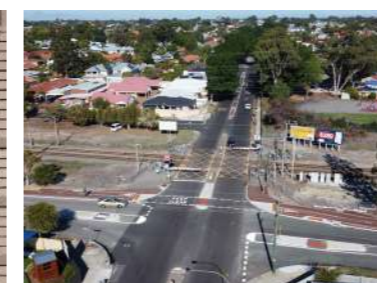
Existing Carlisle Station Level Crossing
