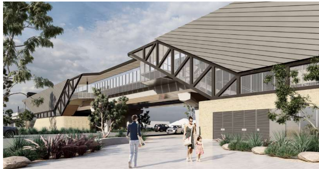
Northern Building Approach
