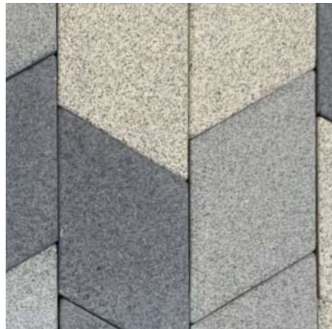
① Plaza Paving
