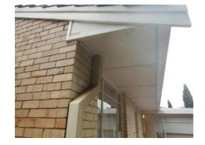
Fibre cement joint cover strips - To eaves lining (61)
