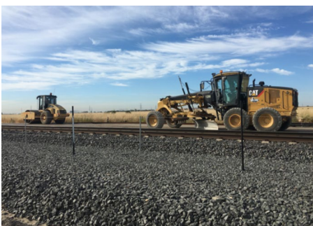
FIGURE 94: GRADER AND ROLLER SPREADING AND COMPACTING CAPPING MATERIAL
