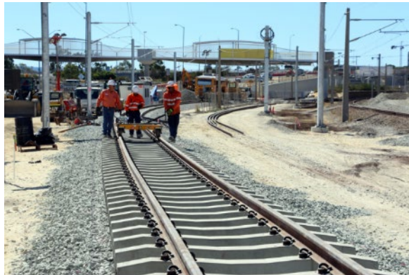
FIGURE 166: THREADING
