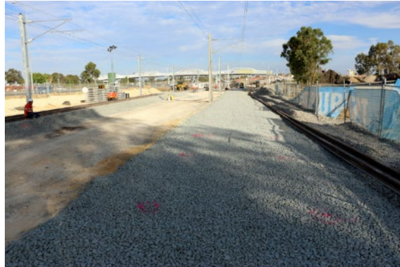
FIGURE 164: BOTTOM BALLAST ROLLED AND READY FOR SLEEPER PLACEMENT
