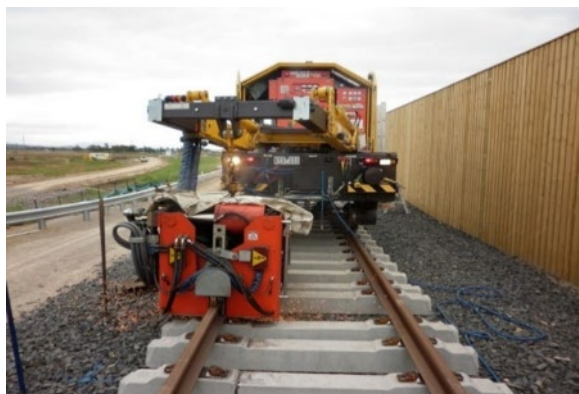
FIGURE 163: MOBILE (HIRAIL) FLASHBUTT WELDER IN OPERATION
