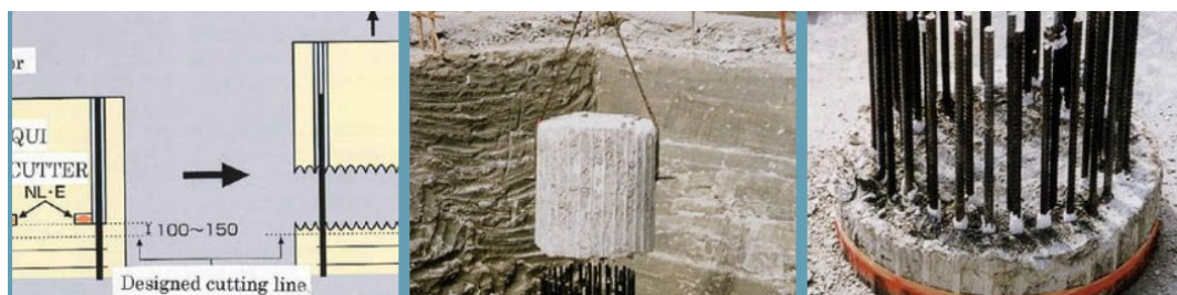
FIGURE 119 PILE CROPPING
