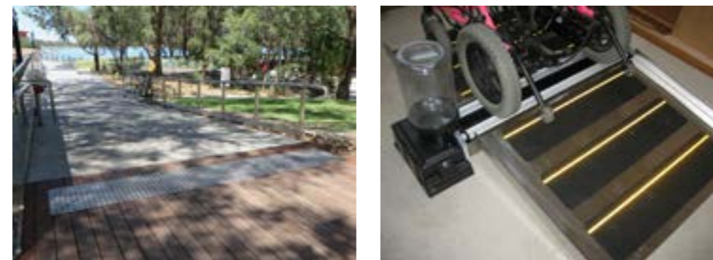
TACTILE GROUND SURFACE INDICATORS TO RAMPS, WHEELCHAIR TYRE WASHING STATION
