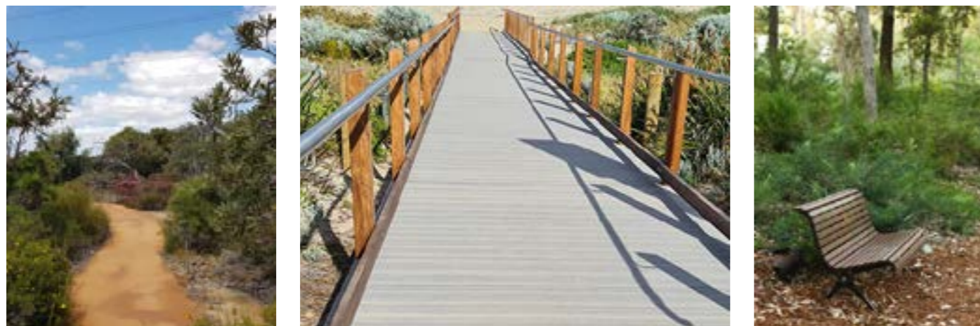
ALL ABILITY ACCESS CLAY ROAD BASE OVERLAID WITH POLY SEALANT / RAMP, VIEW DECKS /LOW KEY FURNITURE
