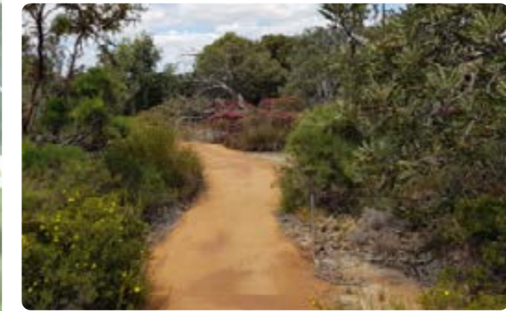
CLAY ROAD BASE OVERLAID WITH POLY SEALANT FOR ALL ABILITY ACCESS
